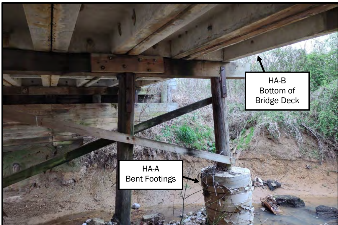
Photo 2: View of HA-A and HA-B on the southern end of the bridge, facing north.
