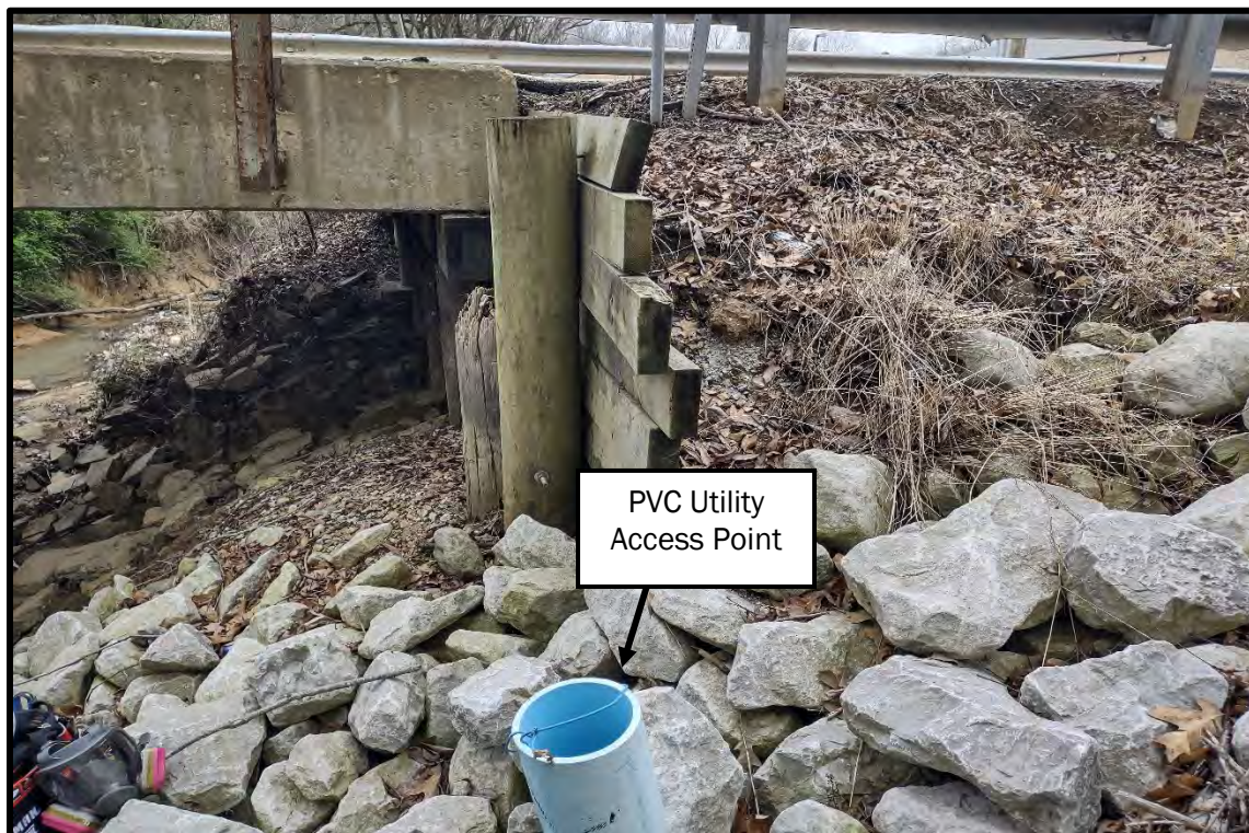
Photo 3: View of access point for a utility conduit comprised of PVC along the southwest corner of the bridge, facing east.
